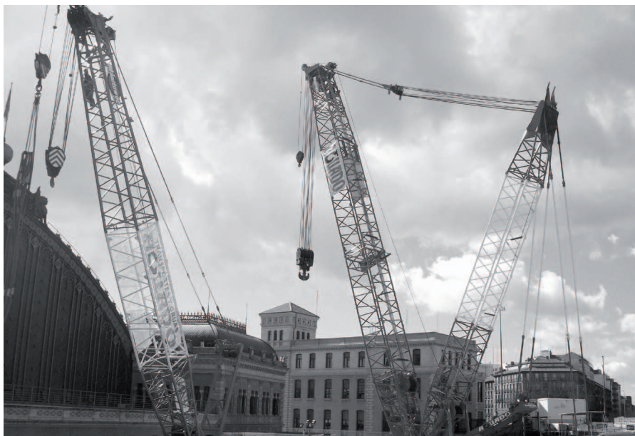
Figure 55 Ropes used for construction cranes
